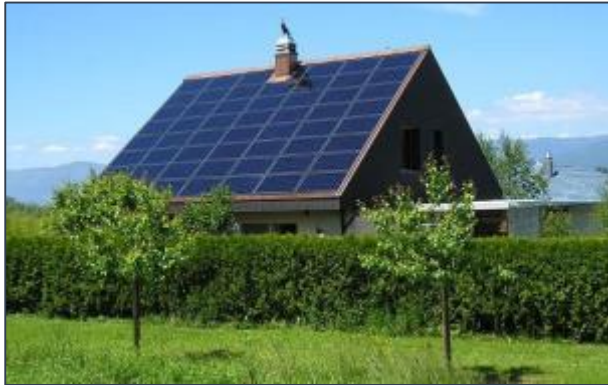
Solar Photovoltaic (PV)
