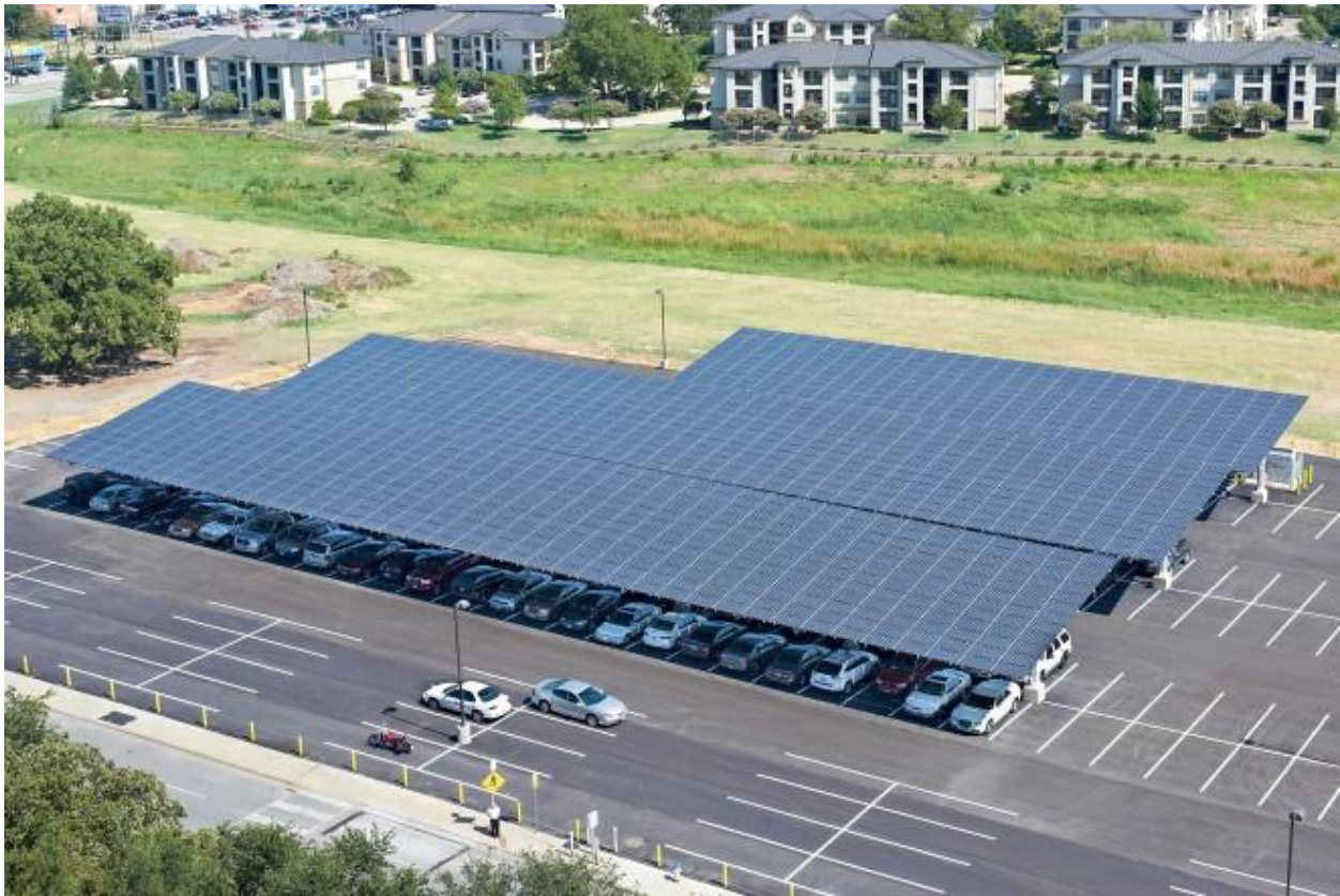
Figure 13. Parking Shade Structures at University of Texas Southwestern Medical Center 43
