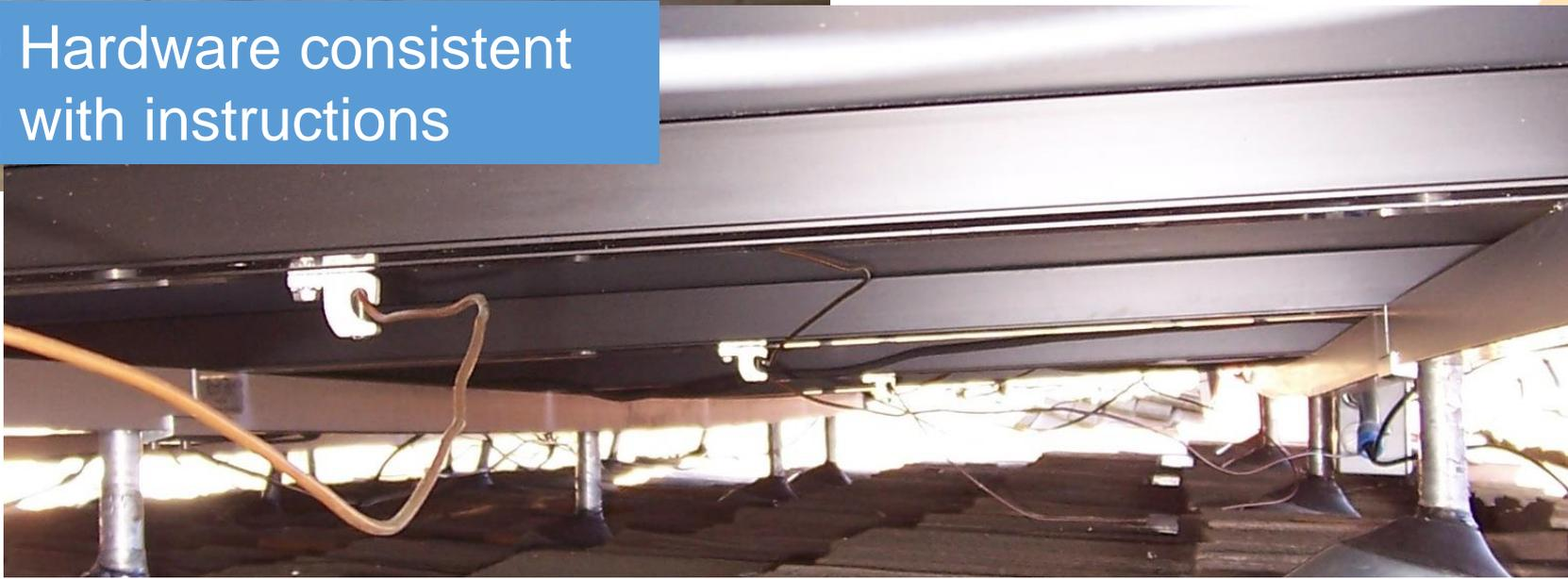
9. Grounding/bonding of rack and modules according to the manufacturer's installation instructions
