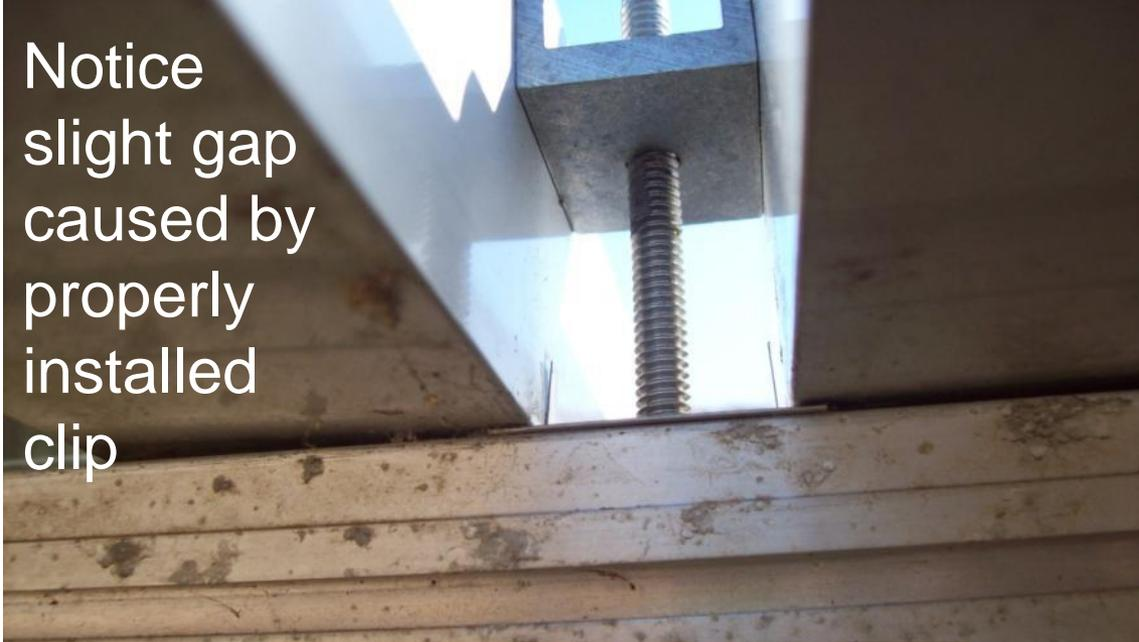
Notice slight gap caused by properly installed clip
